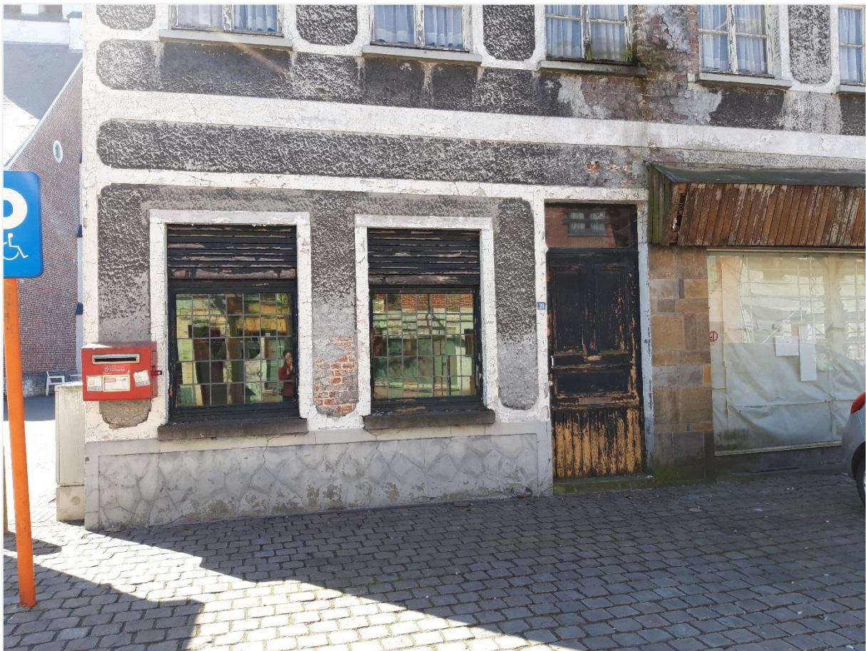
Foto 3: Detail benedenverdieping links
