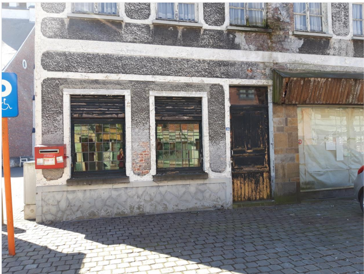
Foto 3: Detail benedenverdieping links
