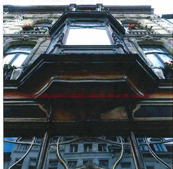
Foto 21: Detail erker in deurtravee.
