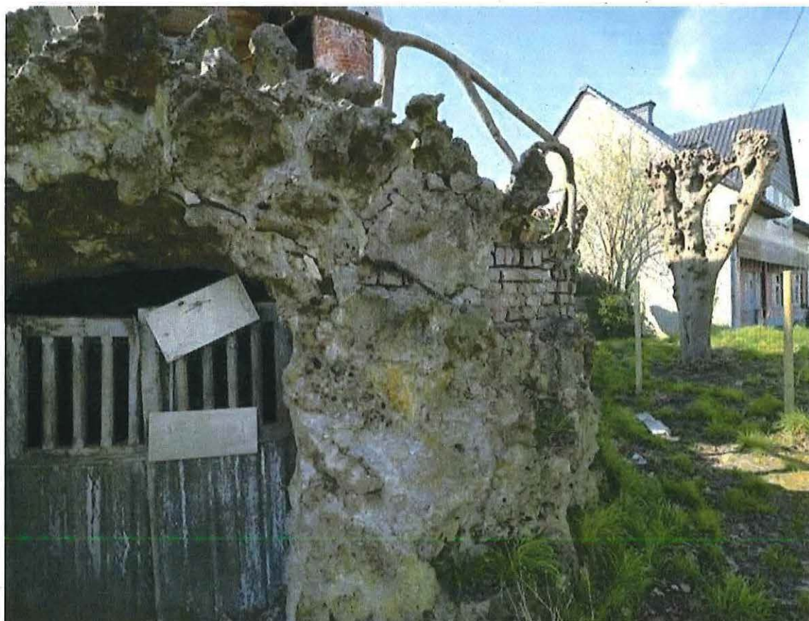
Foto 30: Detail trappenui (© Bressers Architecten 22/11/2017).
