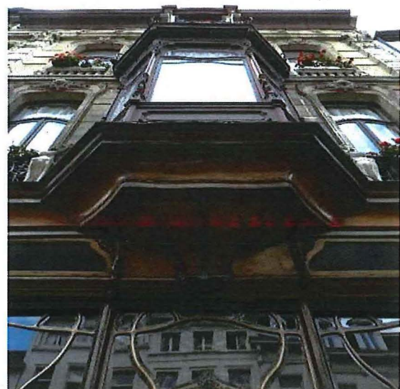
Foto 21: Detail erker in deurtravee.
