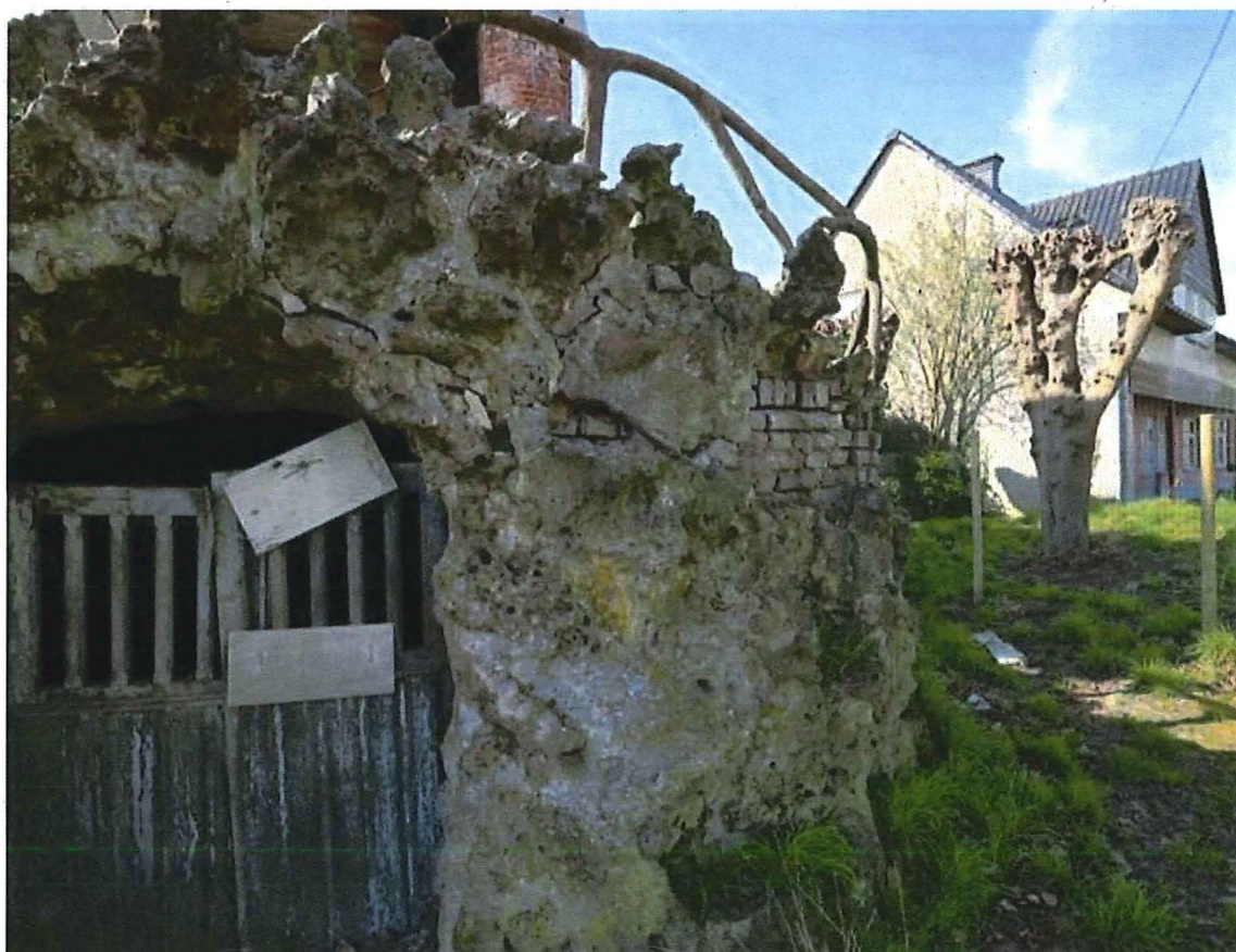
Foto 30: Detail trappenpui (© Bressers Architecten 22/11/2017).
