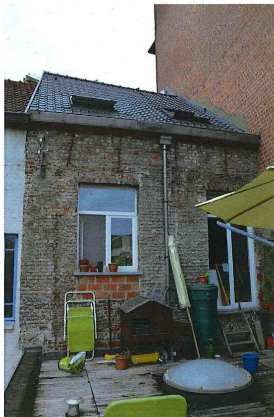
Foto 19: Achtergevel, detail verdieping.
