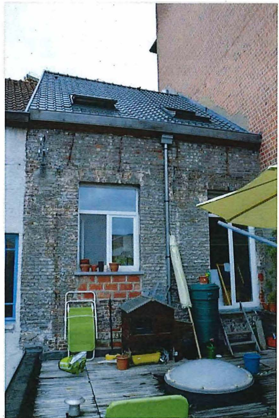
Foto 19: Achtergevel, detail verdieping.
