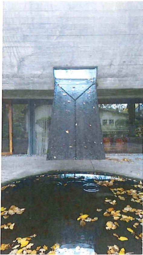
Foto 16: Woning Van Wassenhove. Detail oostgevel. Spuwer.
